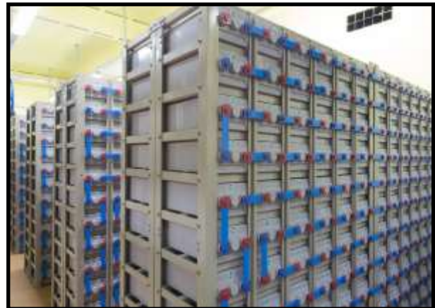
Traditionally, battery modules have been connected by front bus-bars or jumper cables.
