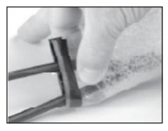
**3.7 Seal Mold.** Starting at bottom of mold, seal and compress sealing mastic around and between each cable to form a resin tight seal.
