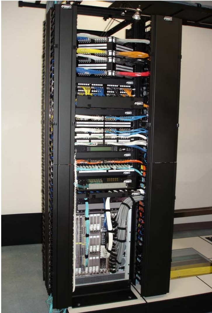
Figure 6. Control centers use standard structured cabling techniques to network the wind farm and communicate upstream.
